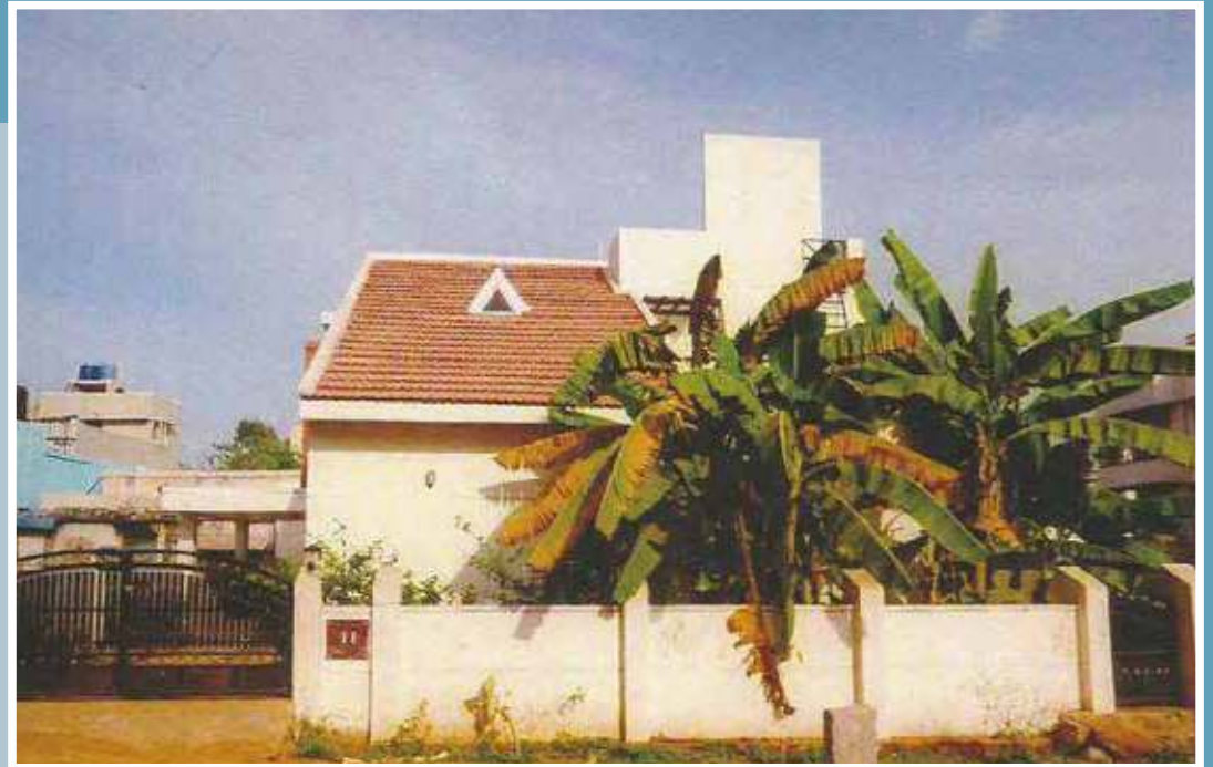
Construction of Residential Building Mr. S. Ravi ( DRDO Scientist ) C.V. Raman Nagar, Bangalore
