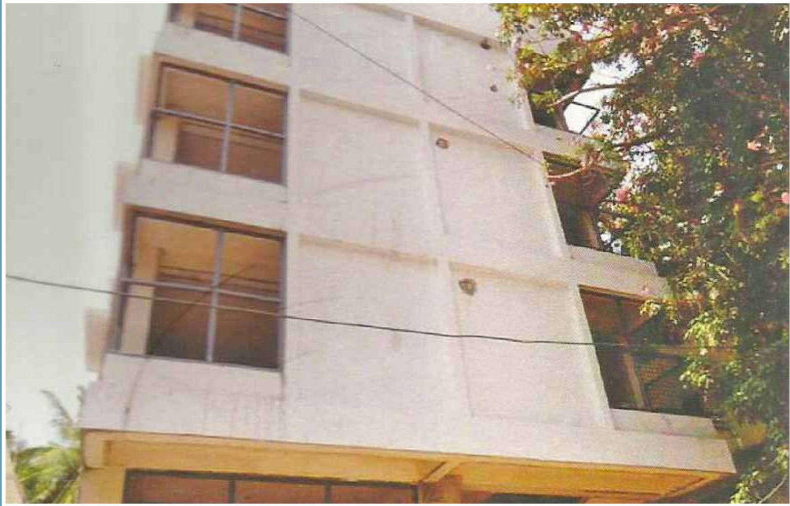
Construction of Commercial Building Mr. Ravi Venkatesh Jayanagar, Bangalore
