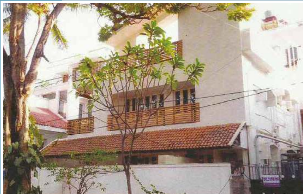
Construction of Residential Building Mr. Sharath Reddy Koramangala, Bangalore
