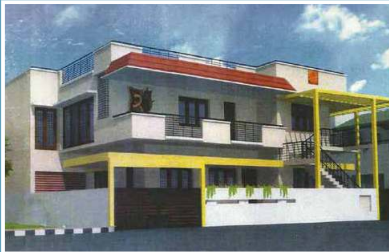
Construction of Residential Building of Mr. Dinesh Chartered Accountant Hanumanthanagar, Bangalore
